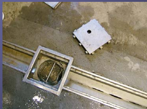
Drain with basket trap inserted
