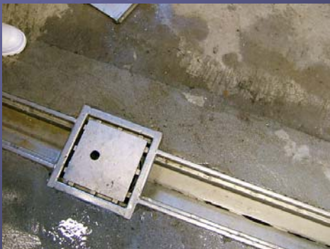
Drain with basket and cover in place
